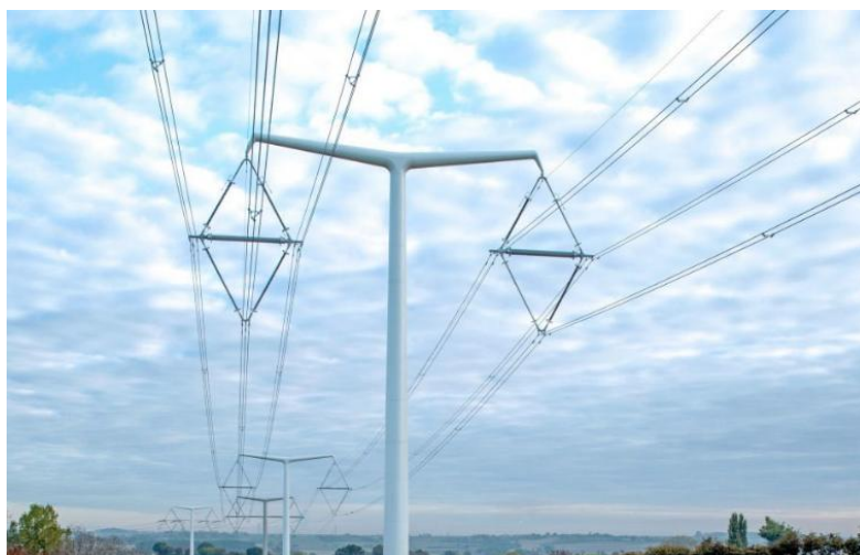
Image 5.9 Typical suspension T-pylon
