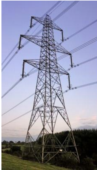
Image 5.10 Typical suspension steel lattice pylon 1
